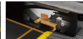
Comb-step Safety Switch (CSS)
