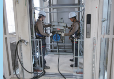
Elevator Installation Training
